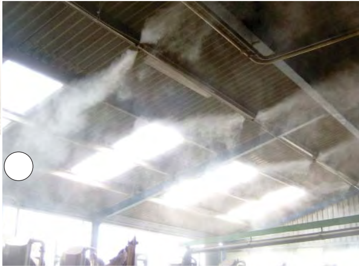
Ivy House Dairy Farm, Milking Parlour
